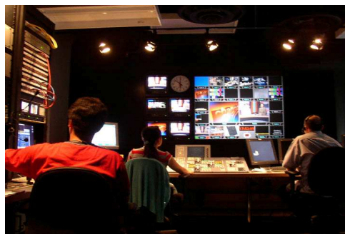
Studio Control Room
